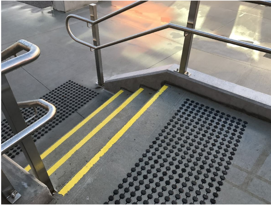
Figure 11: Nosing in the stairs (Source: Luminance Contrast Assessment Tool)
